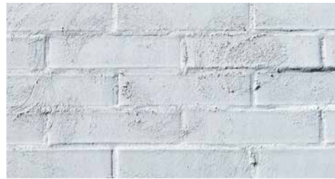
Smooth Stretch 76 mix commons* 290 x 76 x 70mm
