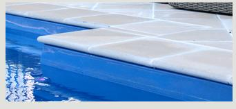
Bullnose pavers are a smooth, rounded edge as an alternative to the standard straight edge.
